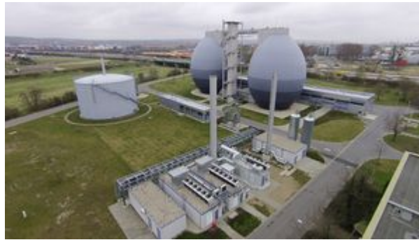
Large sewage works in Germany
