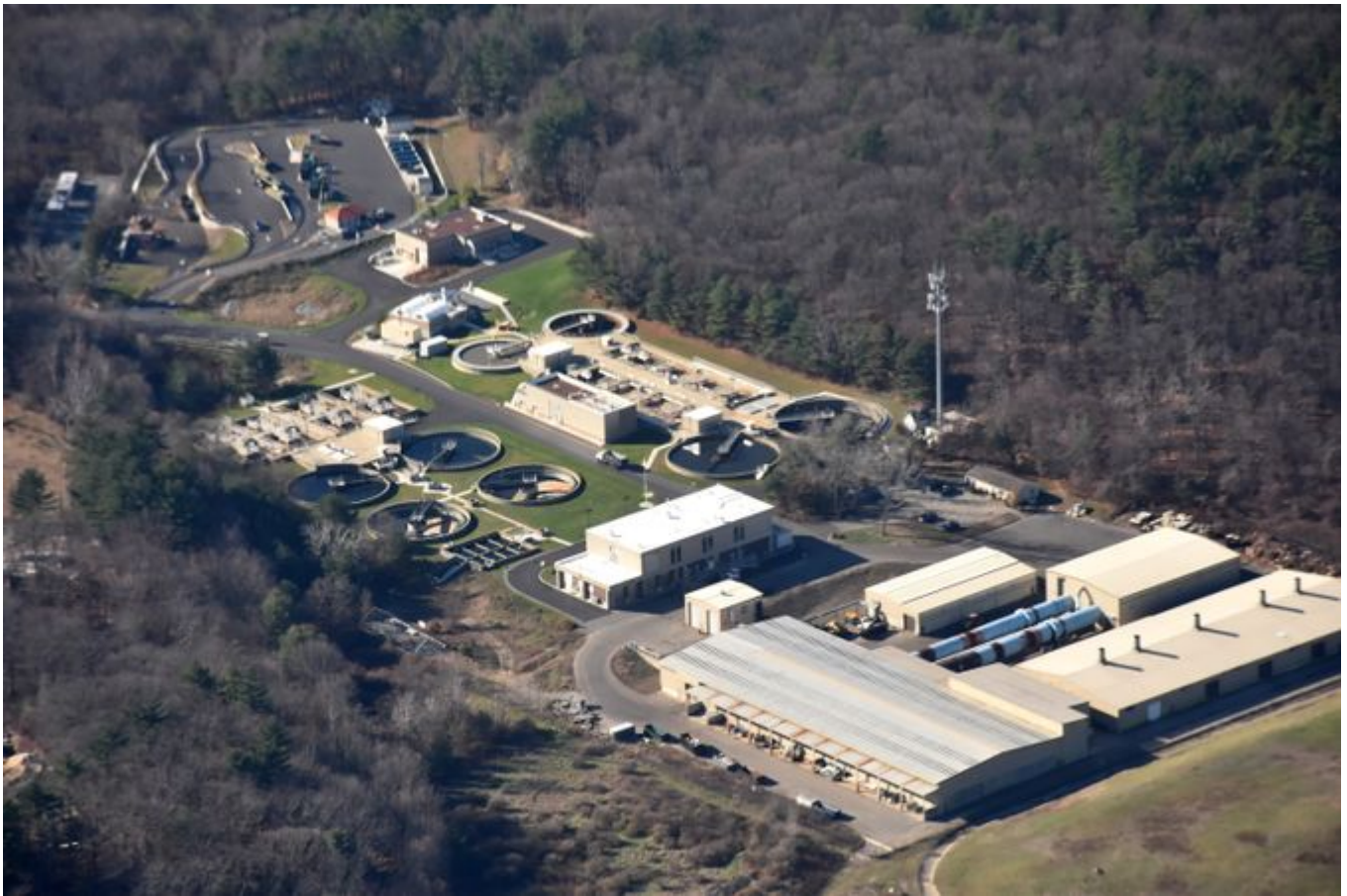
Wastewater treatment plant in Massachusetts , United States
